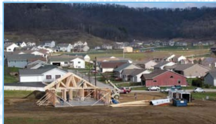
Eco-friendly construction for Messiah Lutheran Church in La Crescent, Minn.
